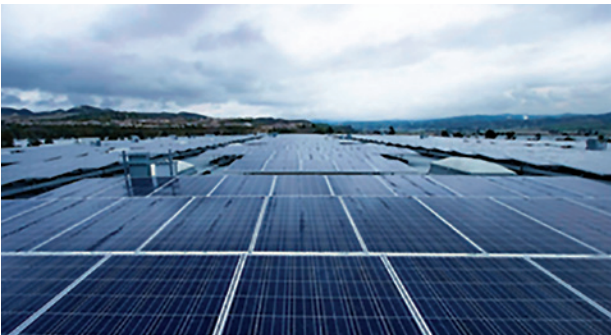
Aerial photo of Hydro Systems facility and its 450 kW solar grid. The grid captures and converts enough energy to sustain the entire operation.
