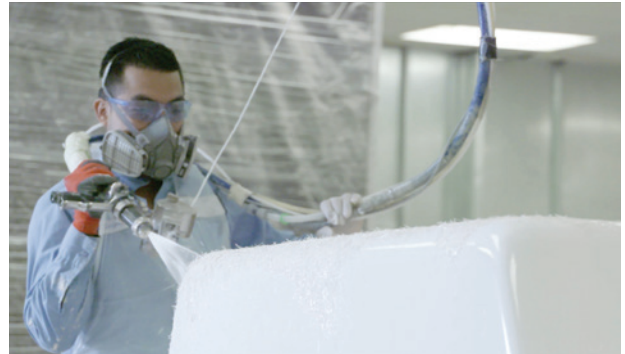
Fiberglass backing applied to acrylic bathtub
