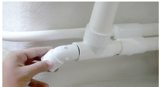
Installation of PVC pipes for whirlpool system
